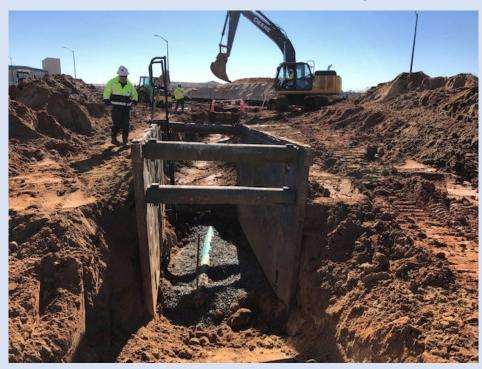
12-inch water transmission line. Construction crews anticipate installing approximately 28,000 linear feet of 12-inch water main during Phase One of the project. Construction is expected to conclude in 2025.
